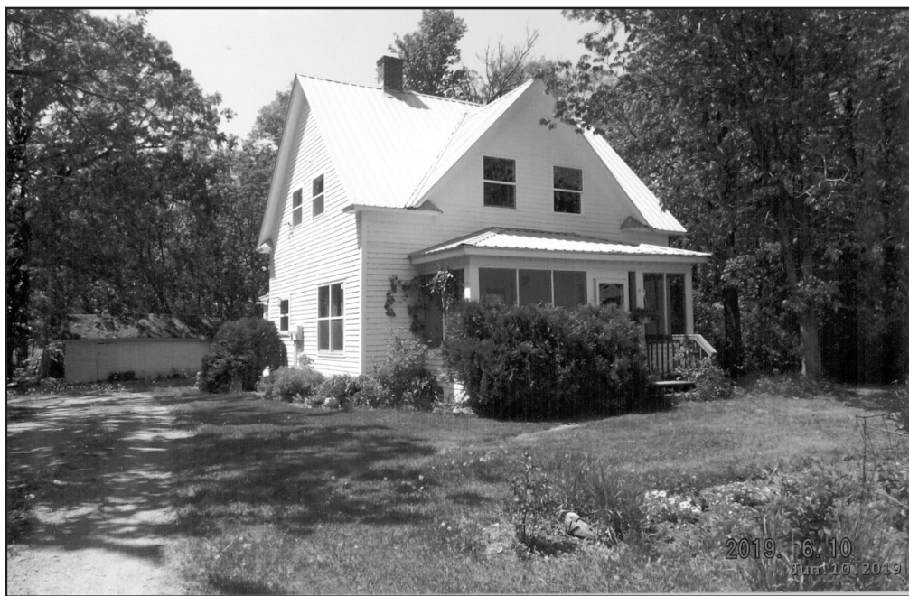
Remodeled Dahlberg home
