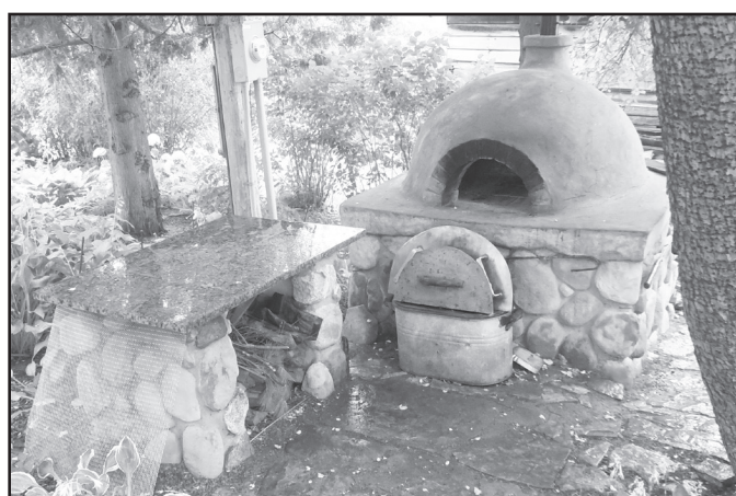
Mary's daughter Annie helped to research and design this clay "cob" oven which they built in the yard with the help of the grandchildren stomping the clay, sand, and straw mix. Mary bakes up to 12 loaves of bread at a time on Fridays and brings them to the Farmers Market in Bagley with an assortment of her homemade jams and pesto sauce.
